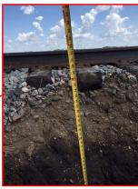
Shows depth of hole created by collapsed drainage culvert.
